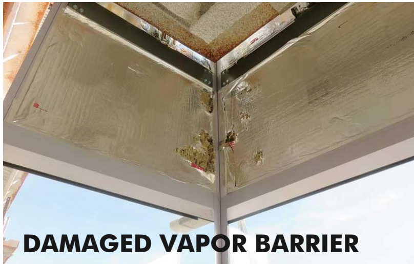
DRIED AND DAMAGED BUTYL
