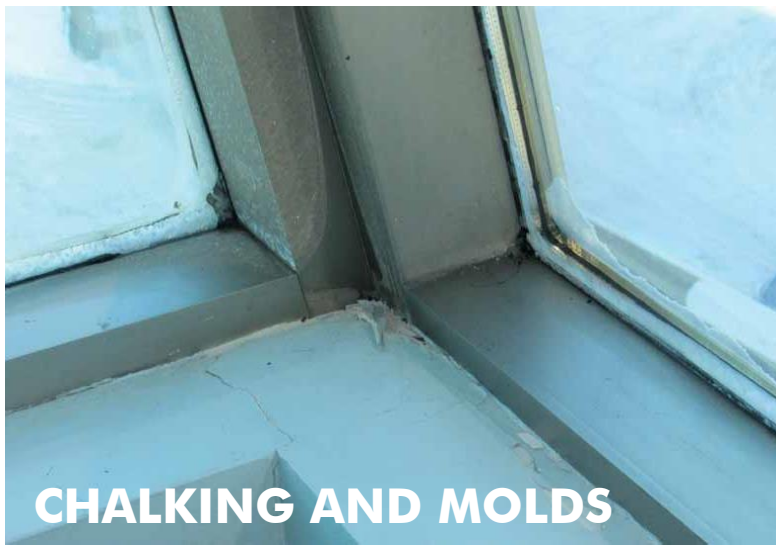
DRIED AND DAMAGED BUTYL
