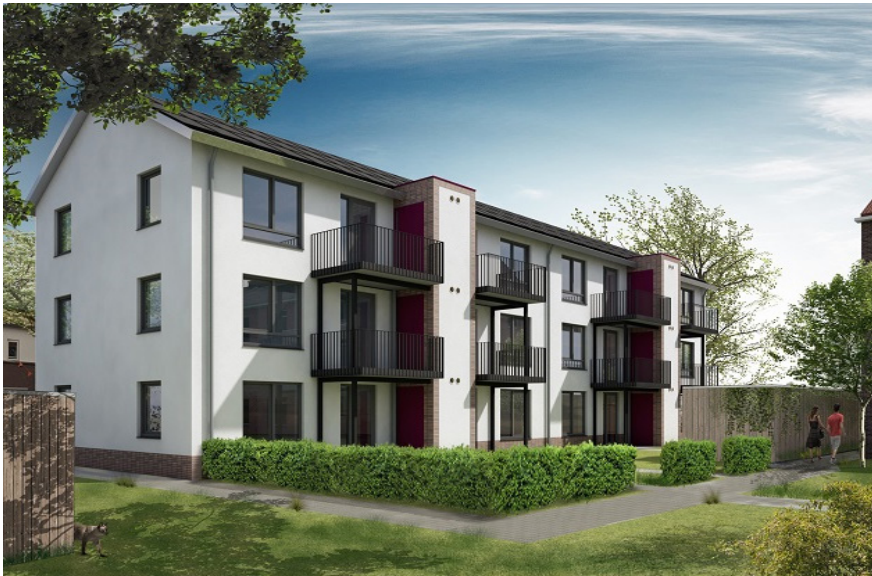
2ndskin demonstrator back side house - After
