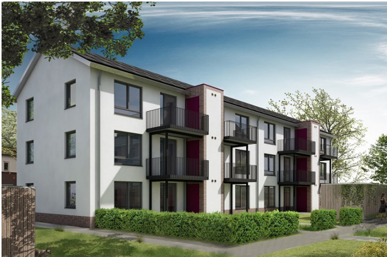
2ndskin demonstrator back facade with installation cupboard
