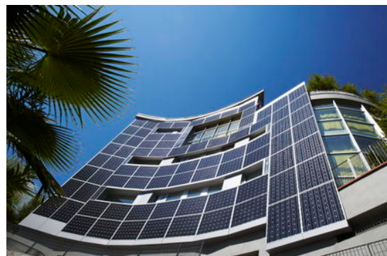
(b) BIPV in a facade structure [15]
