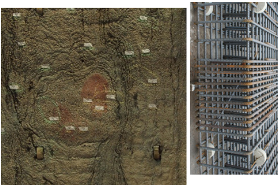
Figure 7. Pattern visible at locations with a strong reinforcement concentration
