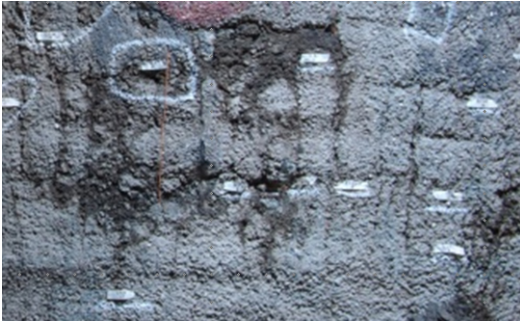
Figure 6. Location of reinforcement bars visible in Panel 2
