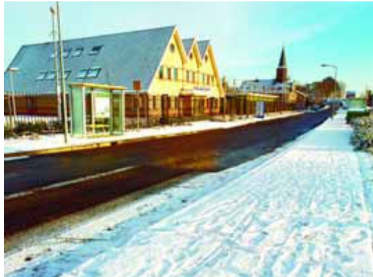
figure A.1-b: a road heated by Road Energy Systems®
