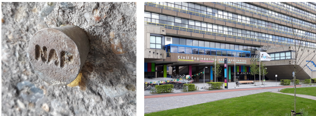
Figure 35.9: Bronze NAP bolt, in a pillar (back row pillar, in the perspective of this photo under the 'C' of Civil Engineering ...), near the B-entrance of the Faculty of Civil Engineering and Geosciences building in Delft. The NAP marker (peilmerk) number is 037E0612, and the given height in NAP is -0.359 m, thus below the NAP reference surface.
