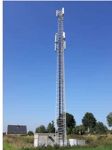
Figure 16.4: A GPS receiver is commonly used to synchronize base stations for telecommunication. Requirements on time-synchronization for this application lie in the order of a \mu\text{s} . The photo shows a base station with a height of 37 m, providing the full range of mobile services from 2G (GSM) to 5G (NR).
