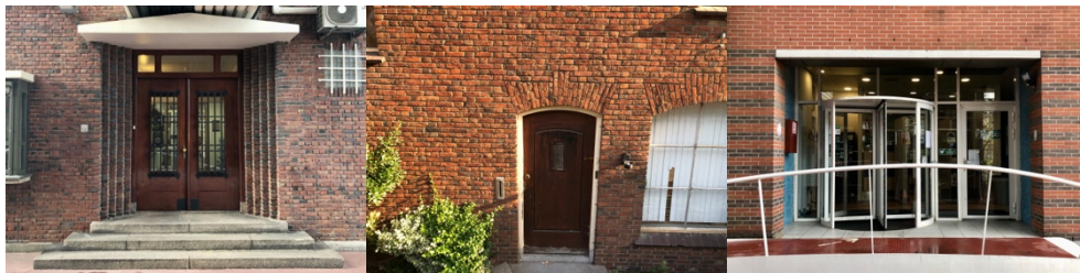
Figure 4. The three entrances of the Harbour Police Station, dating from 1933, 1940 and 1994 respectively, as shown in the case study.
