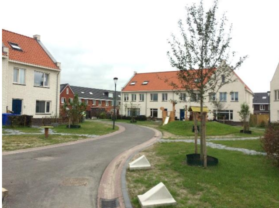
Figure 13. Cycle paths and narrow lanes in RijswijkBuiten (source: own photos)
