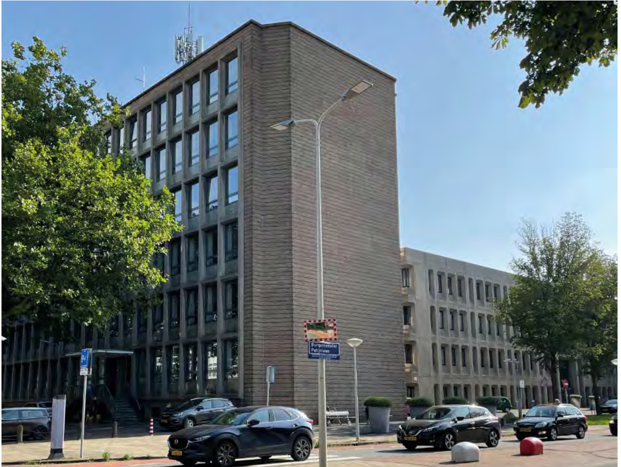
BEFORE - North-east elevations
