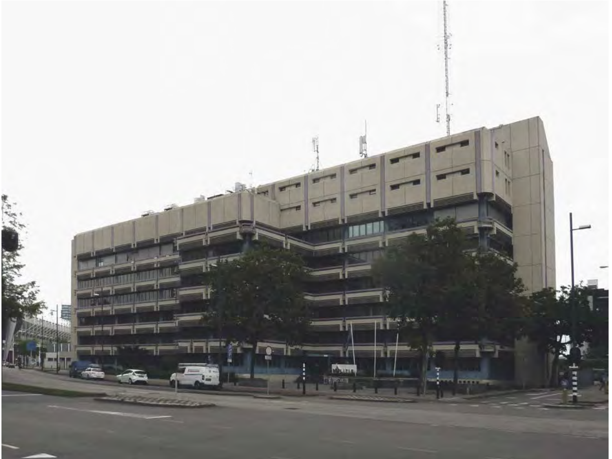
BEFORE - South-east elevation
