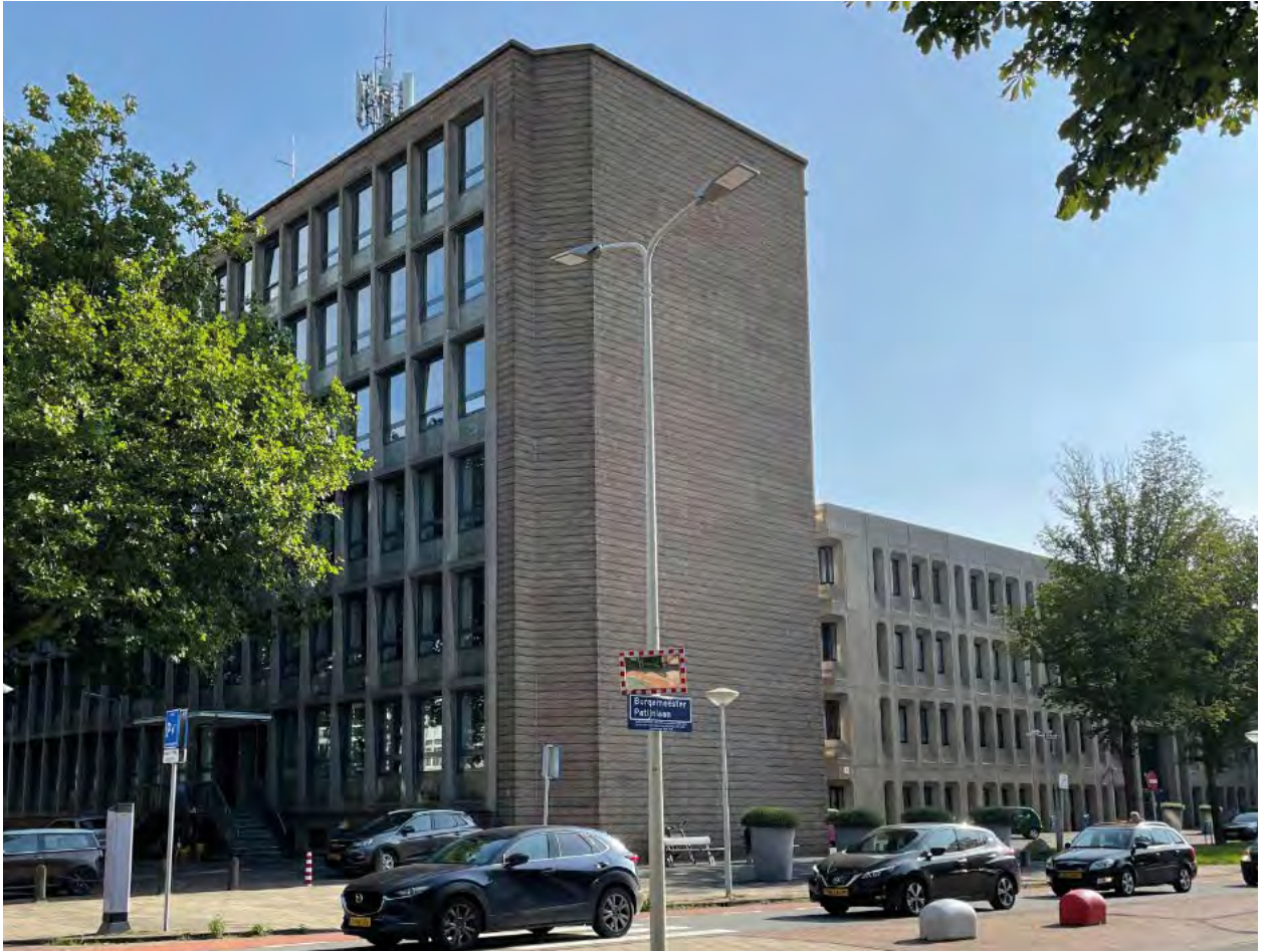
BEFORE - North-east elevations
