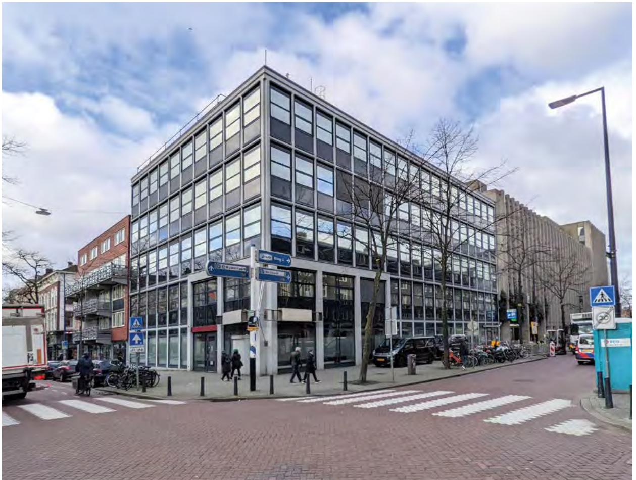
BEFORE - South-east elevations
