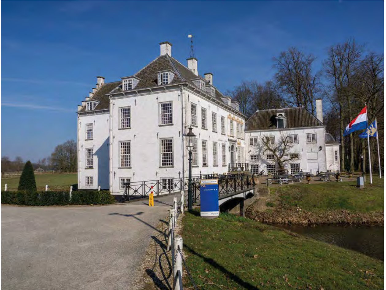
BEFORE - South-east elevations
