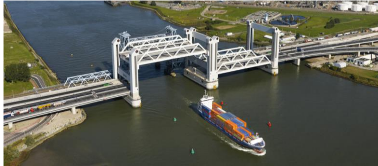
Figure 2.3 Vertical lift bridge, Botlek (NOS, 2015)
