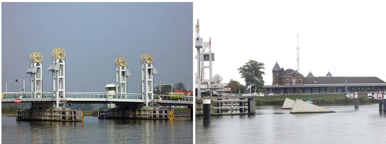
Figure 3.31: Left: City Bridge, Kampen (NL), without concrete ramps (Kampen stadsbrug hefgedeelte by Arend041 is licenced under CC0 1.0); right: with concrete ramps (courtesy Yttje Feddes is licenced under CC BY-NC-SA 4.0).
