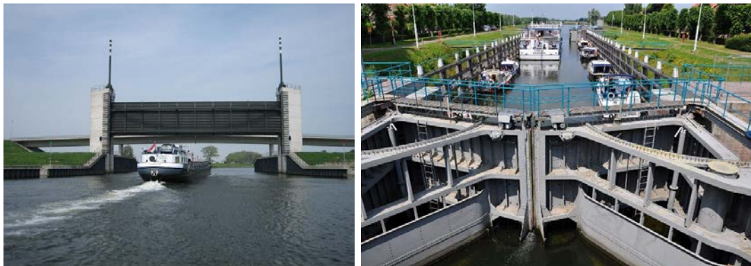
Figure 3.23: Left: Lift lock Kromme Nol near Heusden, Netherlands ( Kromme nolkering 1 by Hullie is licenced under CC BY-SA 3.0); Right: Green lock chamber, Wilhelminasluis near Andel, Netherlands ( Netherlands, Afdamde Maas, Wilhelminasluis by Vincent van Zeijst is licenced under CC BY-SA 3.0).
