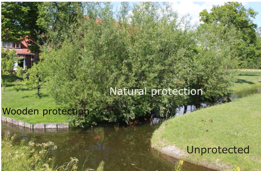
Figure 1.2: Example of current situation in the Netherlands. Canal banks are protected by wooden structures, left unprotected or natural vegetation growing along the banks providing partial protection.
