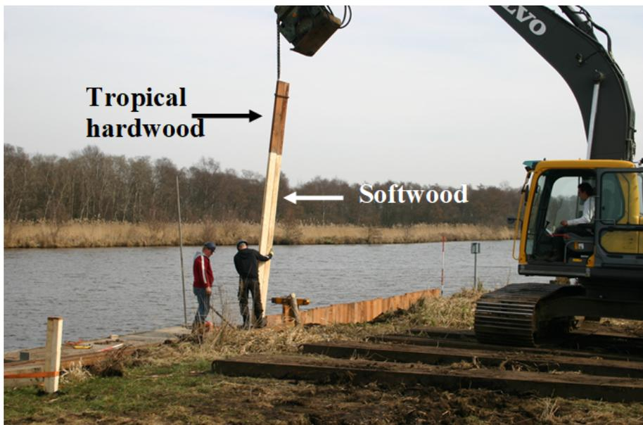
Figure 5.3: Twin-wood sheet pile, combination of tropical hardwood and softwood resulting in improved service life. (Taken from FORECO hout producten. <https://www.foreco.nl/nl/producten/twinwood>)
