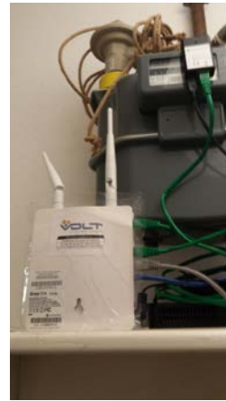
Figure 3.4: Youless electricity meter sensor mounted on a) a new digital meter b) an old gas meter
