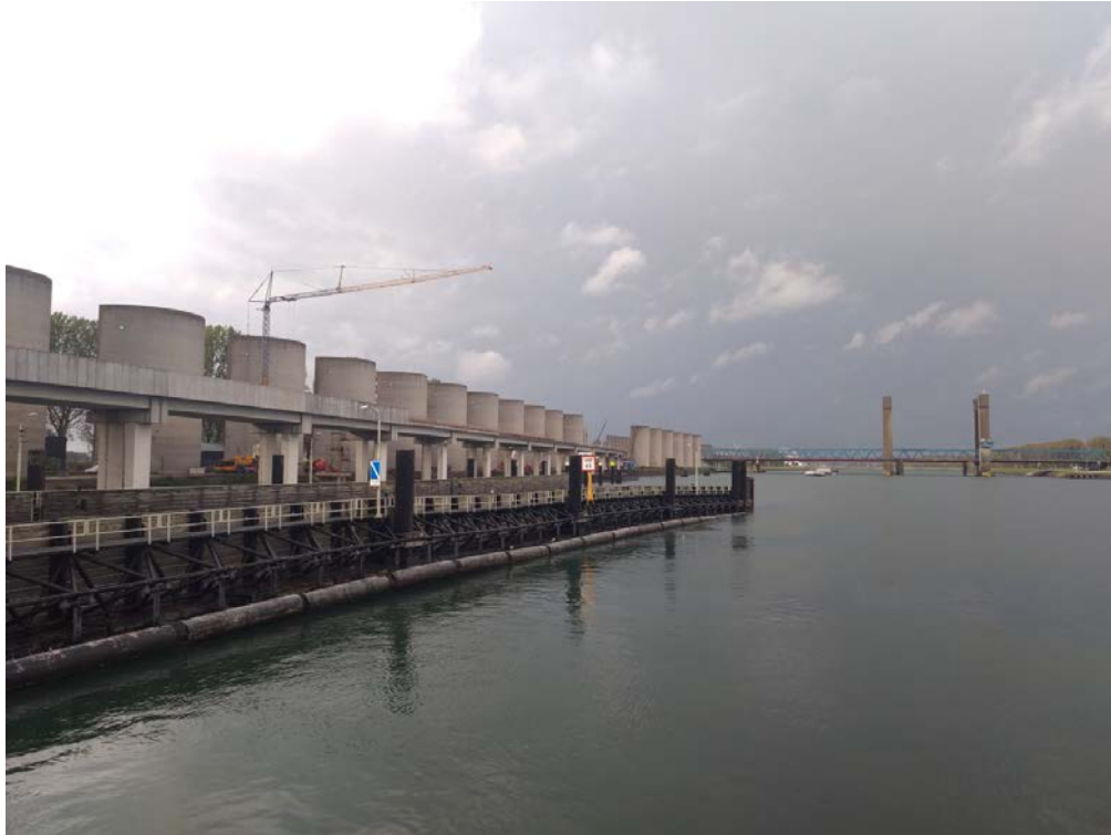
Figure 4.8: Wind screens along the Caland Canal, Port of Rotterdam (by Victor Stoeten is licensed under CC BY-NC-SA 4.0).
