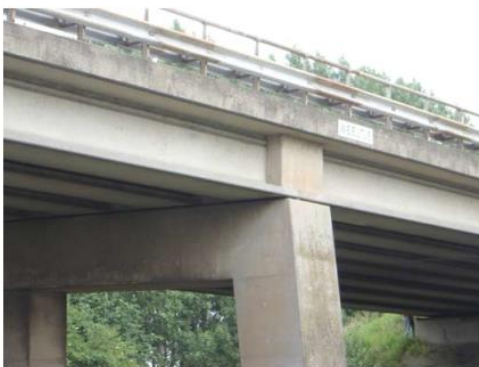
Figure 2.6: Bridge consisting of inverted T-girders [28].
