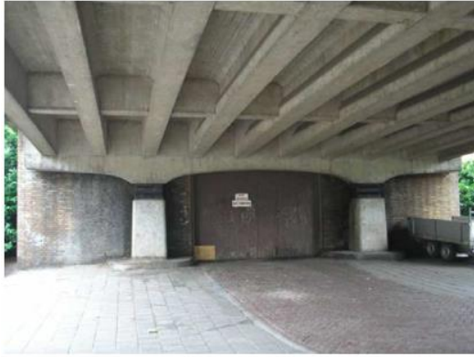
Figure 2.4: Bridge consisting of T-girders with crossbeam in between [28].
