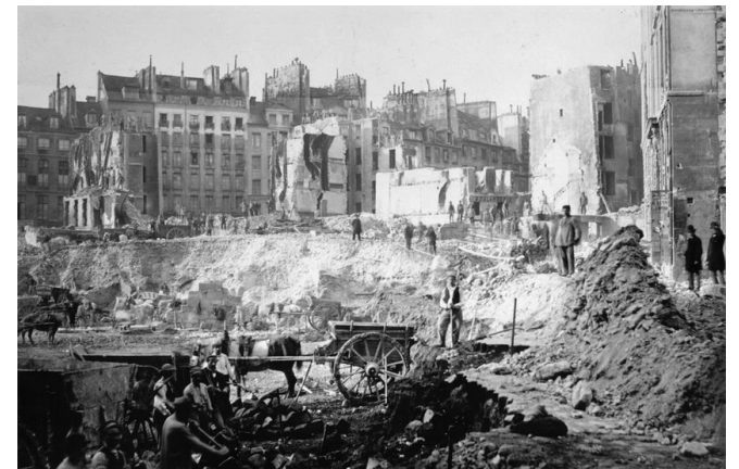
Haussman Renovation Demolition Site BnF (1858)
