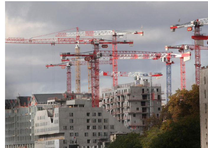
Cranes over New Mix-Use Buildings Olivier Boitet (2018)
