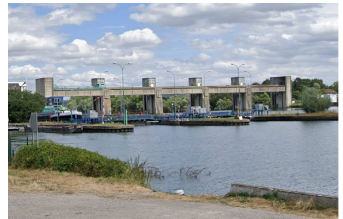
Seine River Dam Screenshot from Google Street View (2021)
