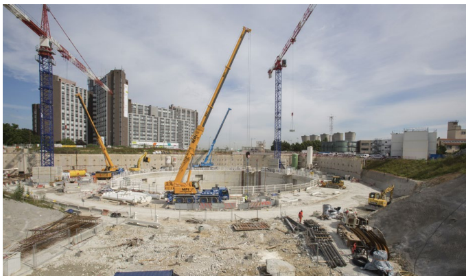
Site of Construction in the Grand Paris BTP (2019)
