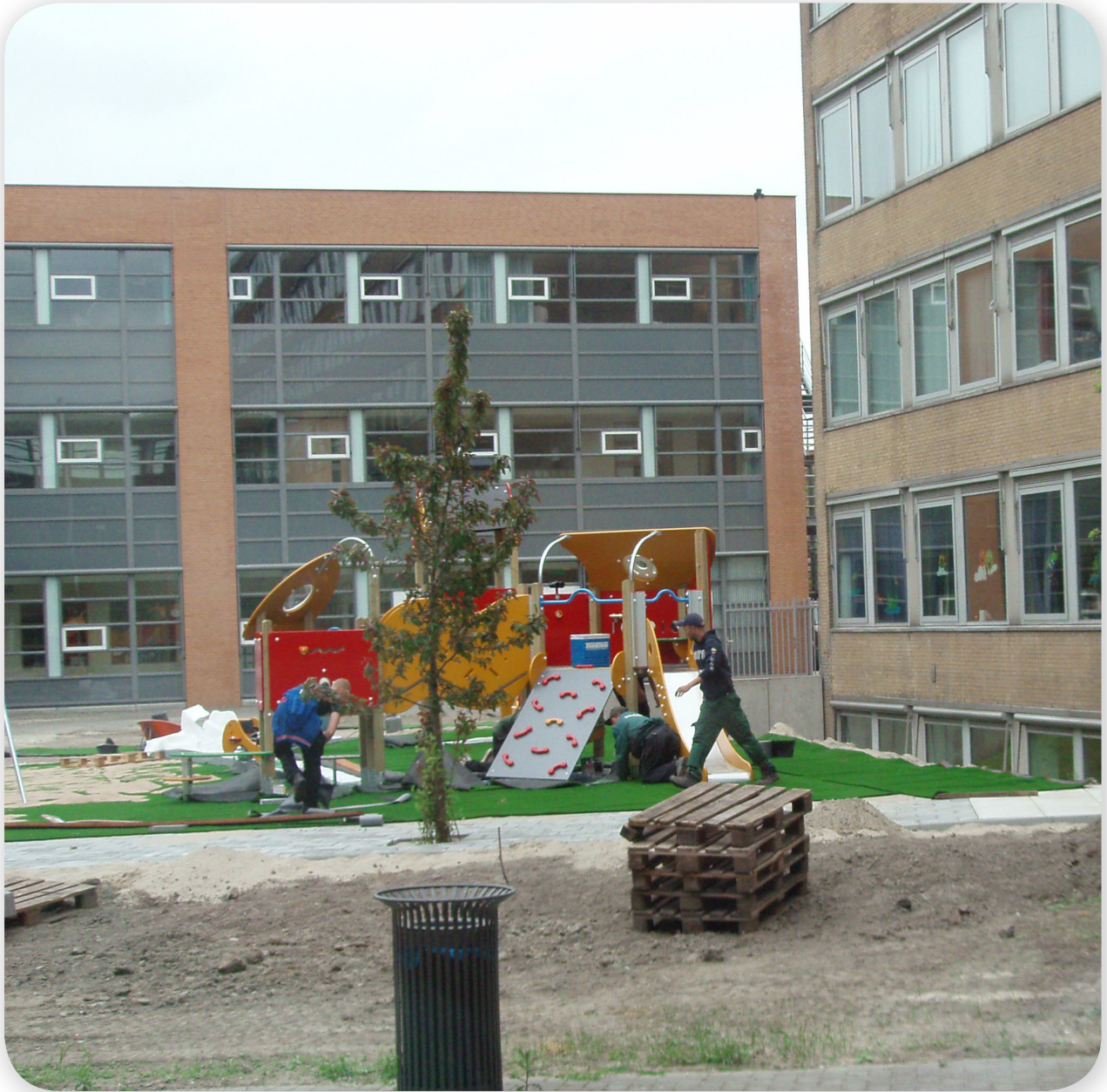
Figure 9. The playground in construction.
