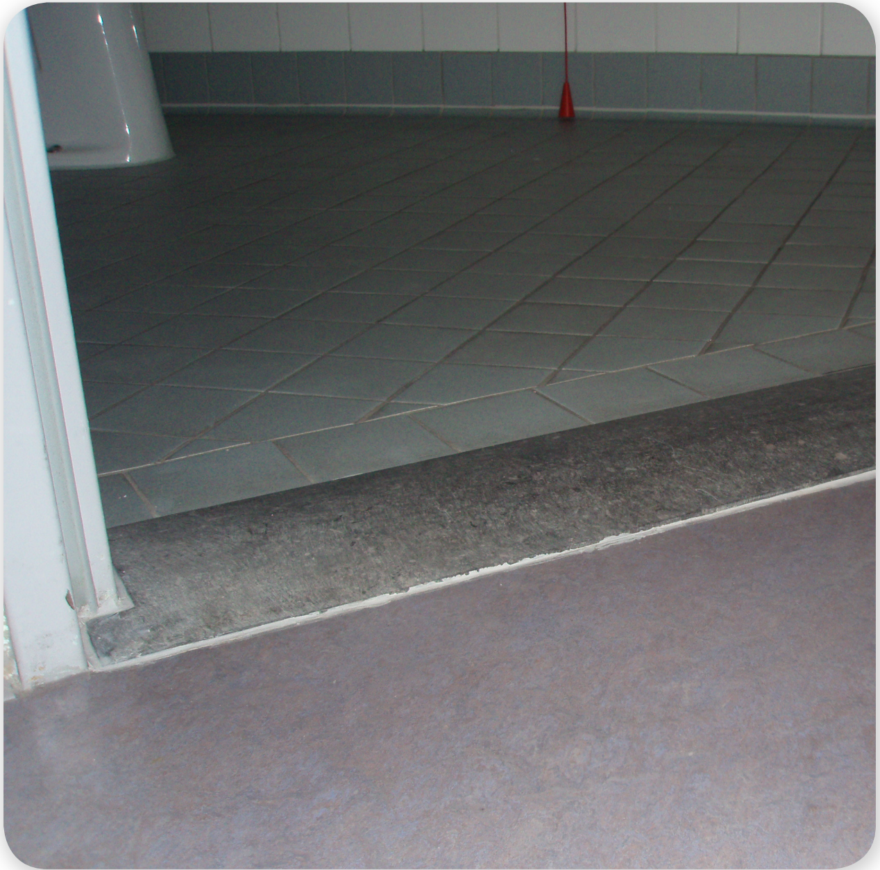
Figure 27. All thresholds and doorsteps had to be flattened.
