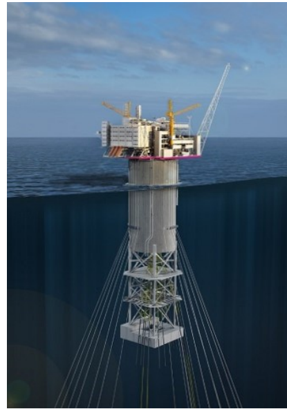
Figure 1.6: A truss spar supporting an oil and gas facility
