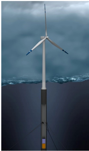
Figure 1.5: Spar-buoy concept supporting a floating wind turbine
