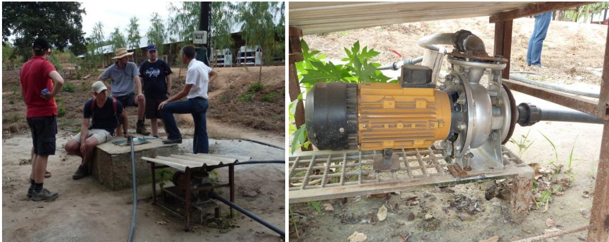
Figure 2.12 Borehole number 7 of Novos Horizontes and the pump used for water transport
