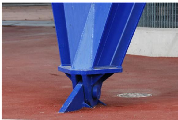
**Figure A-1: Typical 2-1 connection (one part at the foundation, two parts at the column)**
