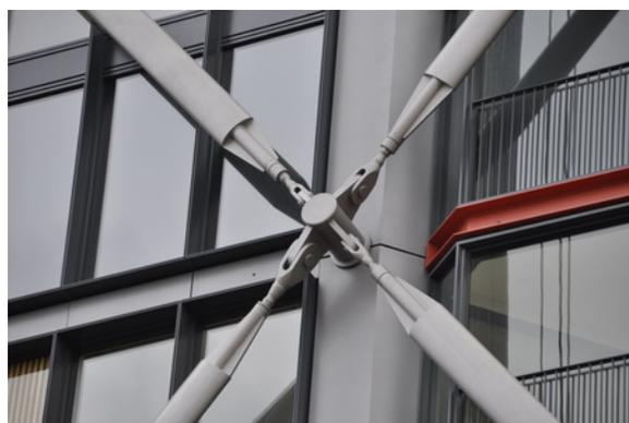
**Figure A-4: Bracing system**
