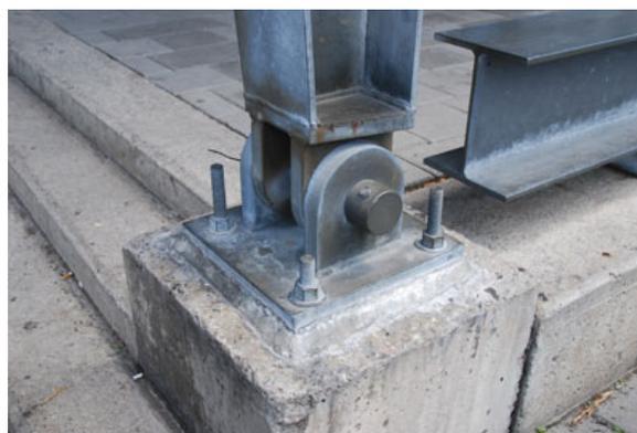
**Figure A-2: Typical 2-2 connection (two parts at the foundation and two parts at the column)**
