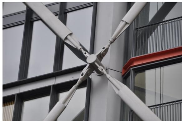
Figure 2-2: Bracing system ([7])
