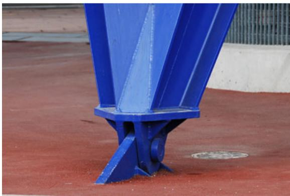
Figure 2-1: Typical 2-1 connection (one part at the foundation, two parts at the column) ([7])
