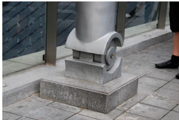
**Figure A-7: Aesthetic connection**
