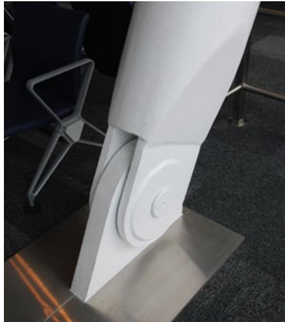
**Figure A-6: Finished pinned member**
