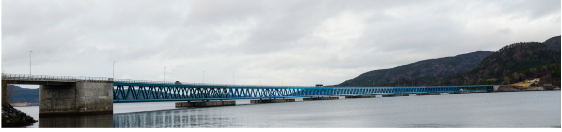
Figure 1: The Bergsøysund Bridge. Photograph: K.A. Kvåle.
