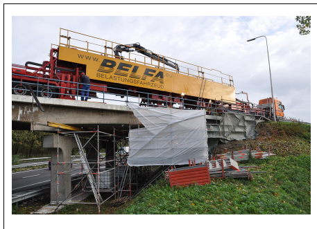
Figure 1. The German BELFA load testing vehicle on the Vlijmen-Oost viaduct in the Netherlands. Reprinted with permission from (1).
