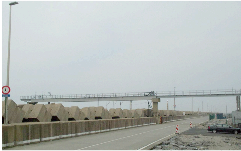
Figure 8. Measurement jetty on the Zeebrugge breakwater
