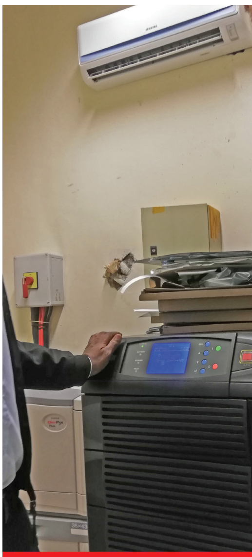
Figure 15. A back-up power supply unit for the CT-scanner in an air-conditioned room. Mbarara Hospital.
