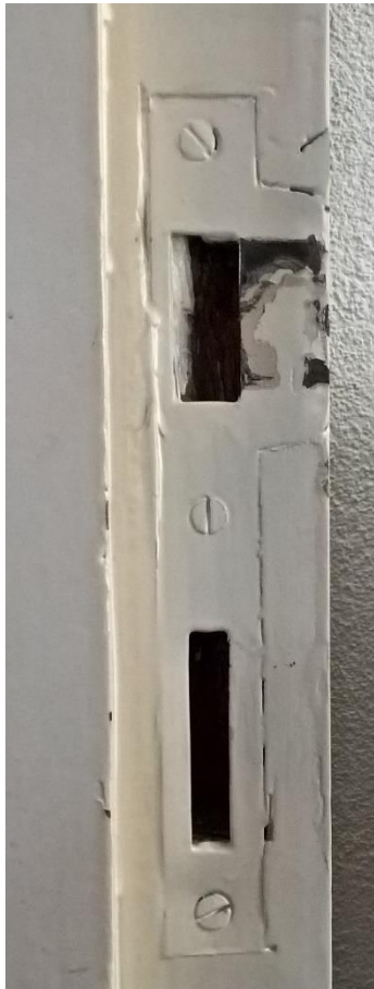
Figure 126 - Steel plate on the wooden door frame
