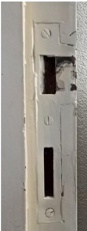
Figure 46 - Steel plate on the wooden door frame
