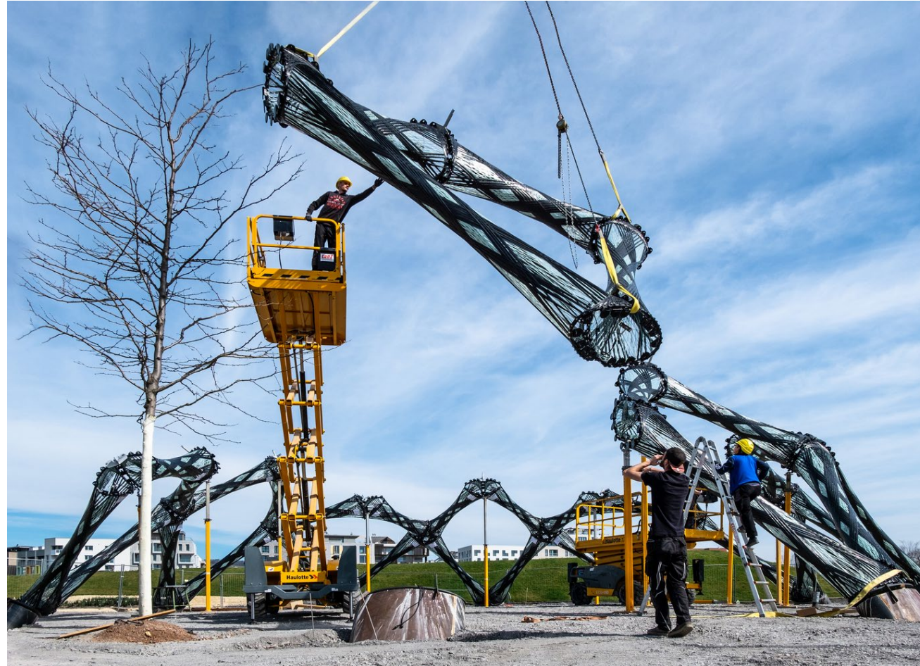
BUGA Fibre Pavilion elements lifted with a small crane
