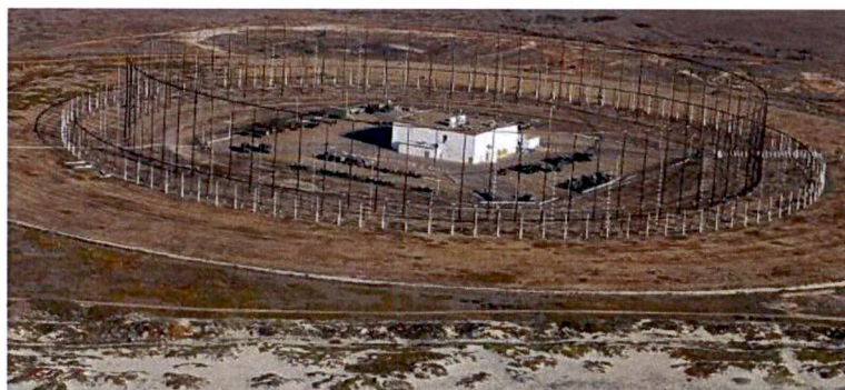
Figure 1.4: Wullenweber antenna, placed at Imperial Beach California in 1964.
