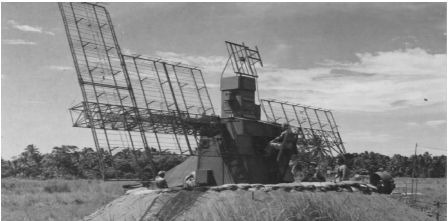
FIGURE 4.1: An SCR-268 at Henderson Field, Guadalcanal [61]
