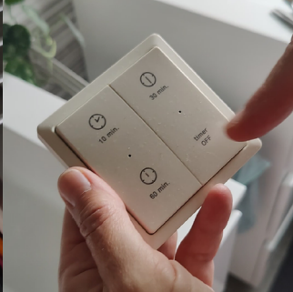
Figure 6: Ventilation control in bathroom
