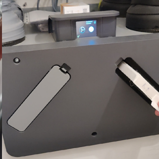
Figure 7: Change the filter
