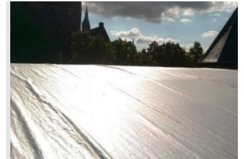
figure 7.9: translucent/reflective summer cover of the Prinsenhof to prevent excessive heat. Photo: Octatube
