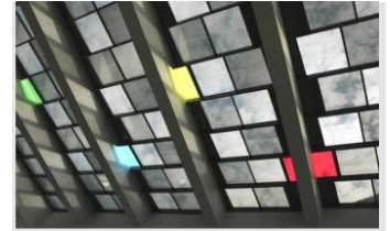
figure 5.3: Bejar market in Spain; semi-transparent, integrated PV in a glass roof (Yang & Athienitis, 2016, p. 888).
