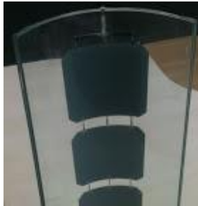
figure 5.18: 'regular' crystalline silicon laminated in a double glazed module (Casini, 2016, pp. 329, 331)
