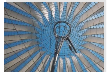
figure 4.8: glare prevention (and acoustical improvement) with textile blinds (Wurm, 2007, p. 124)
