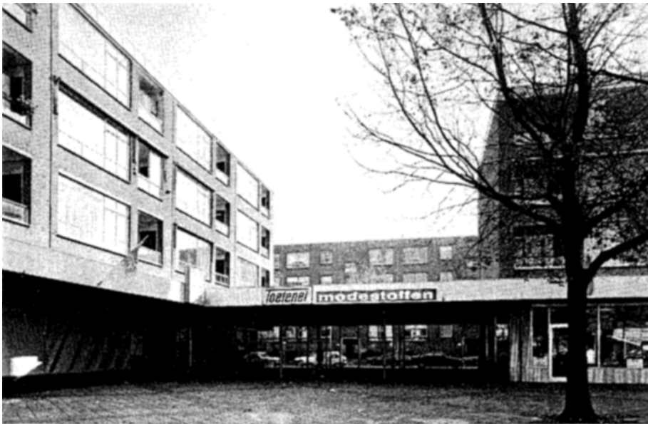
Figure 5 The De Stede estate is an example of a typical 1960s residential district with dwellings above shops. The estate contains both the district shopping centre and a tower block with 84 balcony-accessed dwellings (13 storeys) and 30 balcony-accessed flats in 3 storeys built above shops. Along the edges 116 staircase-accessed dwellings are situated. In total this location comprises 230 dwellings and 13 shop premises.
