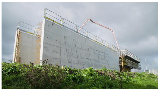
Figure 8. Full scale demonstrator in situ cast self-healing concrete water reservoir, Hoogvliet, The Netherlands.
