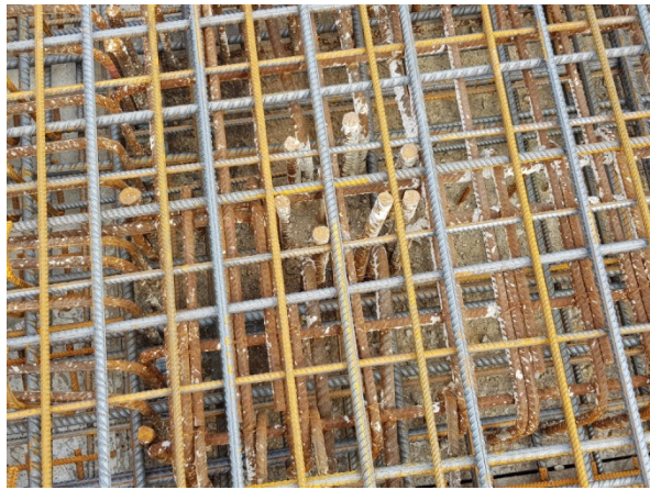
Figure 4. Picture of a finely meshed reinforcement network for watertight concrete constructions impeding easy casting of concrete.
