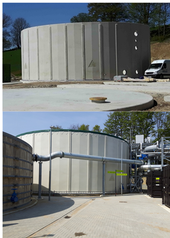
Figure 7. Prefabricated wastewater treatment tank under construction (top image) and in service (bottom image). Prefab elements bearing the triangular logo contain self-healing agent while the other, reference elements, do not.
