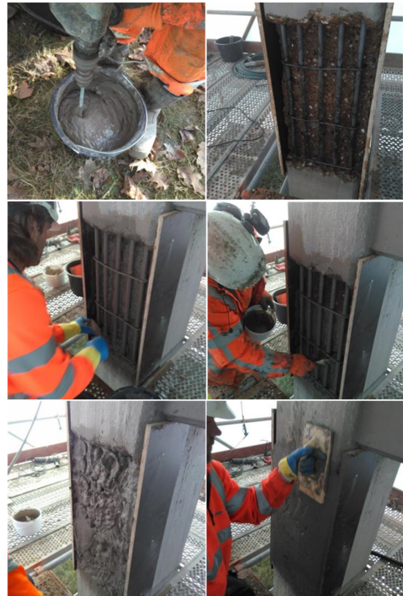
Figure 5. On site structural repair of damaged steel reinforced concrete column with bacteria-based self-healing repair mortar.
