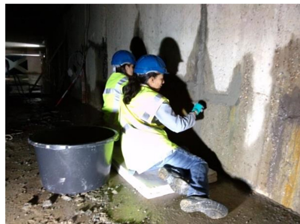
Figure 6. Manual repair of actively leaking cracked concrete basement walls using bacteria-based self-healing repair mortar.
