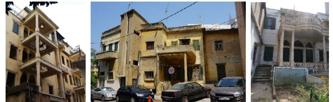
Figure 3.7: Abandoned housing in Mar Mikhael (NAHNOO, 2020)
