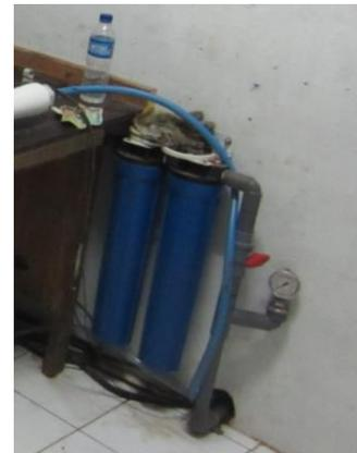
Figure 7.6: Pre-filters, system shut-off valve and inlet pressure gauge.
