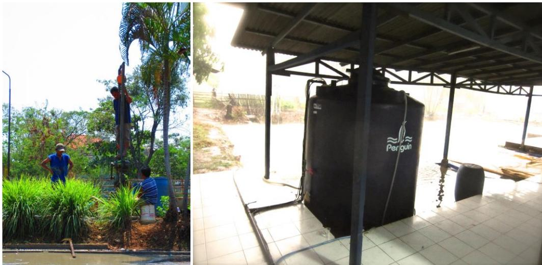
Figure 7.3: On the left the well during construction, and on the right the reservoir eventually used.
