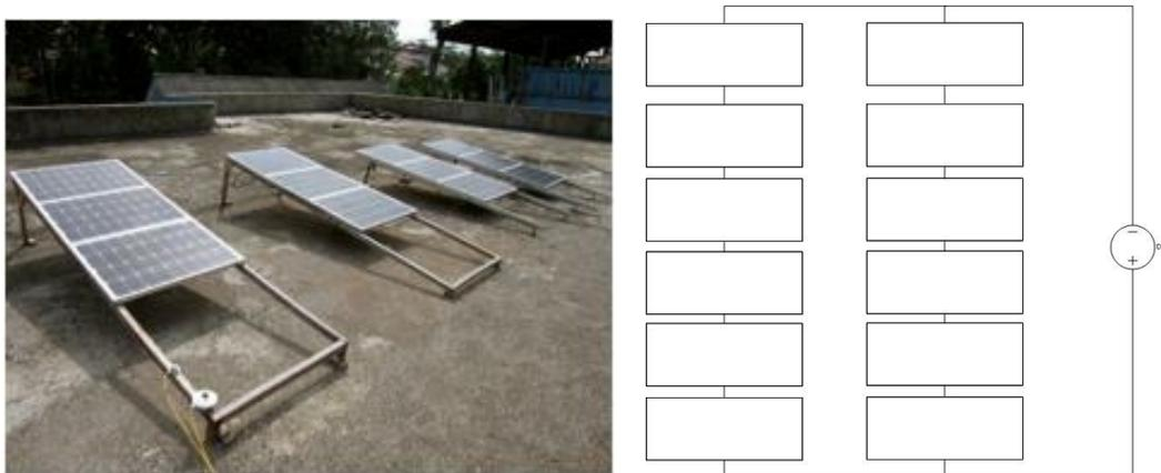
Figure 7.4: PV panels installed on the roof and their configuration.
