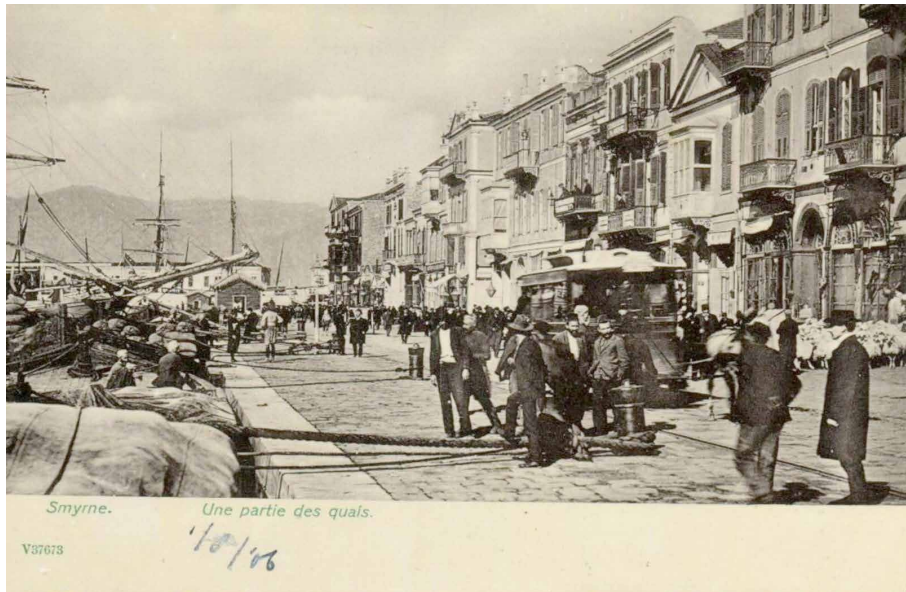
FIG. 6.7 A Part of the Quay (courtesy Mehmet Sunucu).
