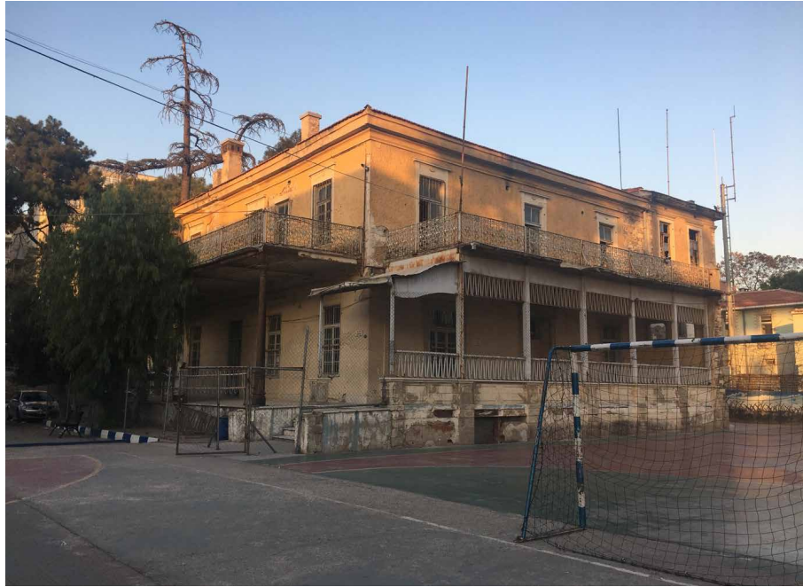
FIG. 7.11 Abandoned Richard Whittall Mansion located in the property of a high school (Fatma Tanış).
