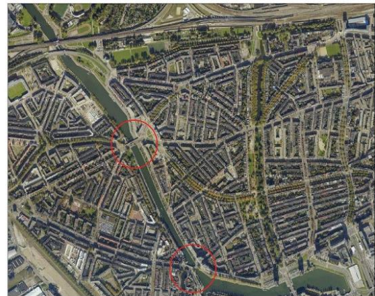
The two bridges that connect Het Nieuwe Westen with neighbourhood on the west
