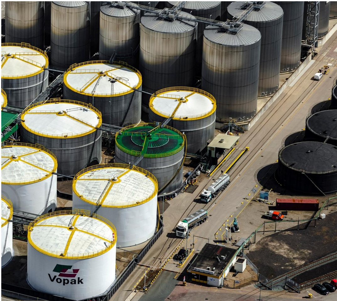
(b) Close up of Tanks at Vopak Terminal Vlaardingen [99]. Photo taken at location of star in Figure B.2a.
