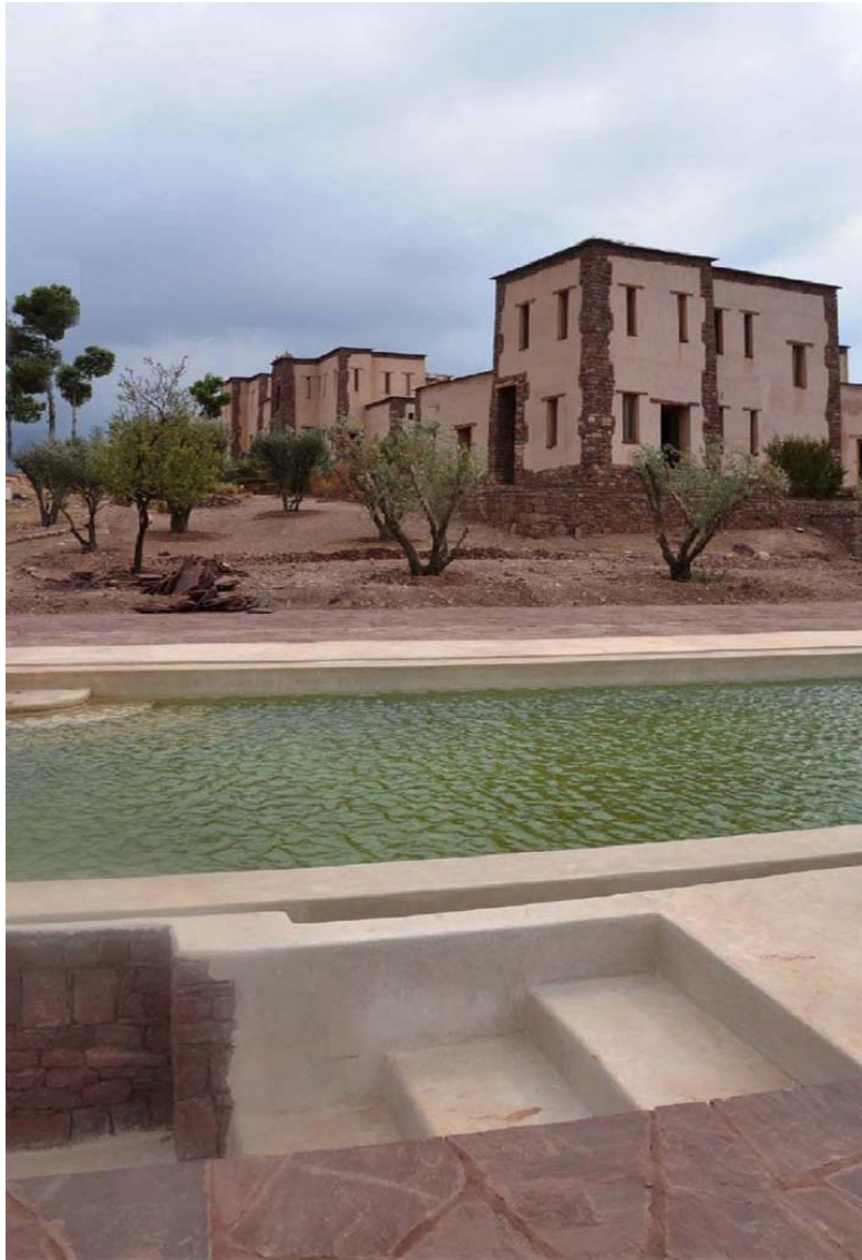
Ksar Akkal, 2012, Salima Naji This spa complex is found in a Berber village in the Atlas mountains, near Marrakech. The construction and materials are based on vernacular Berber building methods and are one with the context. Naji is an influential Moroccan architect with a regionalist view on architecture, respecting local culture and building methods without use of modern principles.
