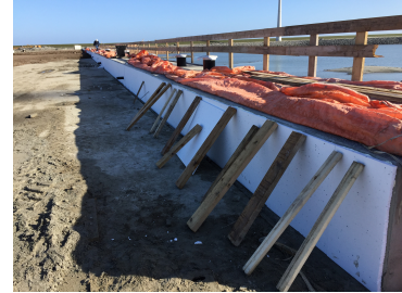
Figure 5.8: EPS elements during construction of the relieving platform
