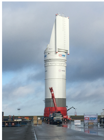
Figure 2.7: Assembling of the NMS 8800 in December 2017 (Groningen Seaports, n.d.)
