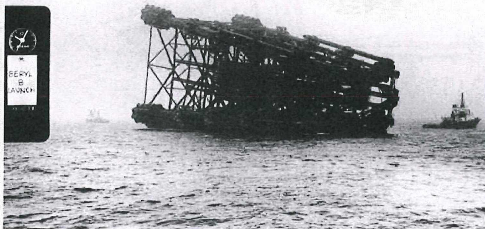
Figure 2. The BERYL B jacket before the launch.
