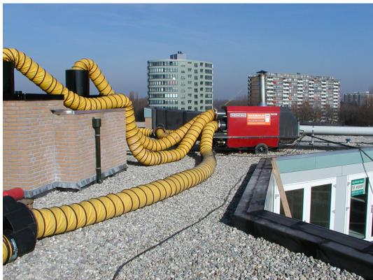
Figure 2.2: The mobile/movable system having multiple hoses is showcased. As can be seen, it has two cavities on the left side through which more hoses are connected. The system is placed on the top of the building which shows it is totally outside the place from where a heating effect is needed.
