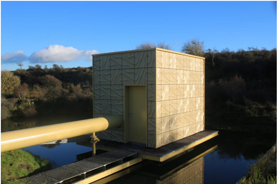
Figure 5.3.: Façade panels applied at the pumping station in a natural reserve [picture from D1.9 WIDER UPTAKE report].
