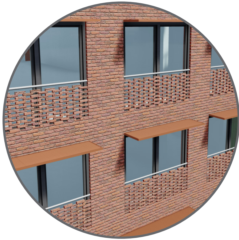
Permanent brise-soleil shading on the facade
