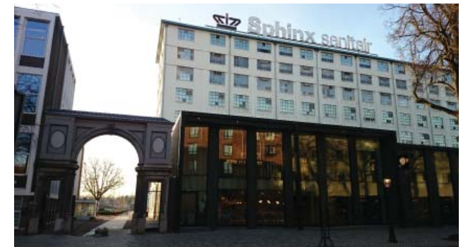
Figure 16. The “Eiffel” one of the industrial buildings from the former Sphinx factory, present day
