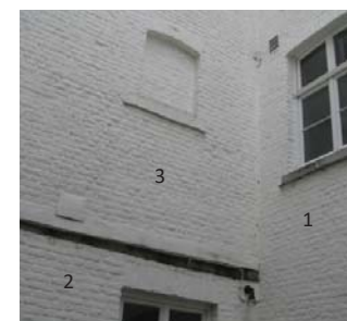
Figure 127. From the small outdoor area different building periods can be seen
