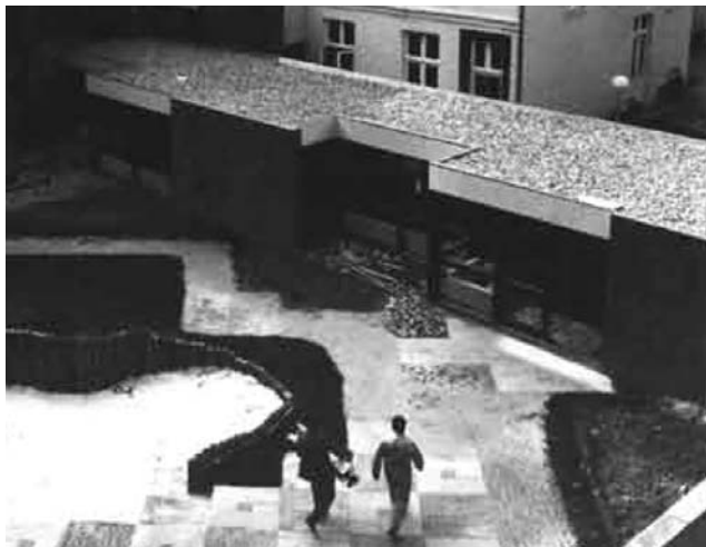
Figure 53. The new entrance hall that divides the courtyard
