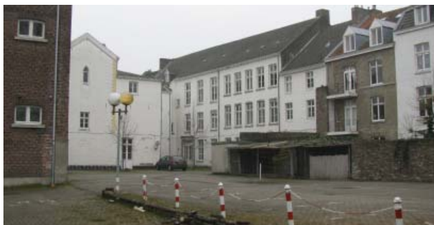
Figure 100. First courtyard, seen from the parking lot
