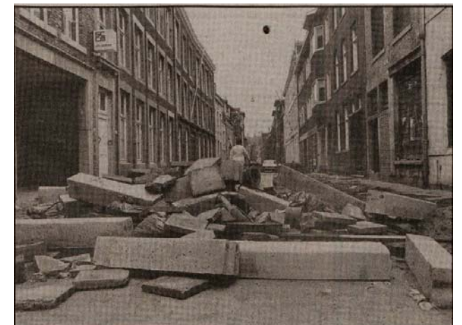
Figure 52. Damage after the squatters had a farewell party
