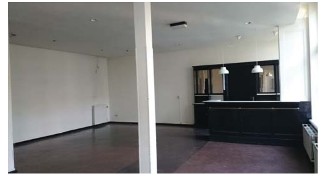
Figure 91. Ground floor of the houses along the Capucijnenstraat
