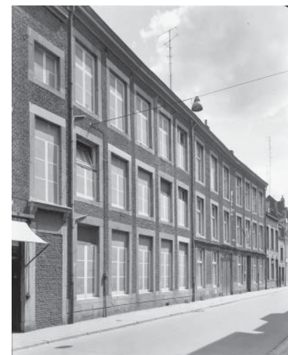
Figure 115. Front façade of the Miséricorde complex, 1962
