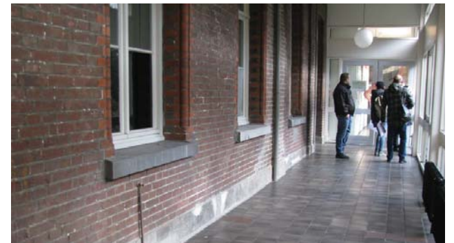
Figure 92. Beneath the concrete balcony from 1926
