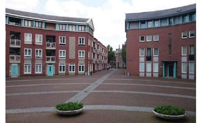
Figure 97. The Miséricorde plein, away from the complex
