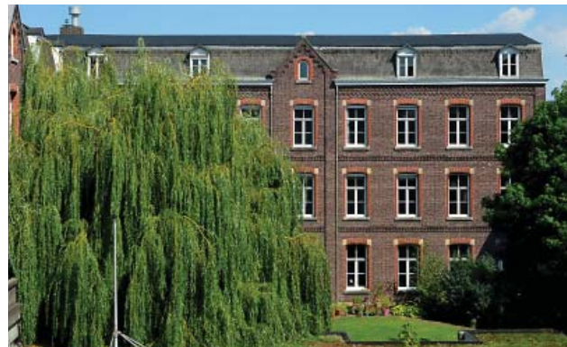
Figure 79. Front side from the Laundry and ironing wing
