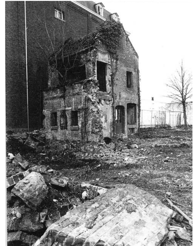
Figure 55. The pavilion before restoration
