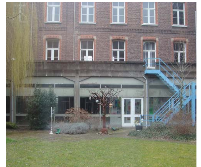
Figure 141. The concrete balcony seen from the inner courtyard
