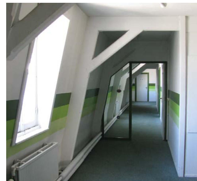
Figure 136. A part of the roof structure of the Laundry wing
