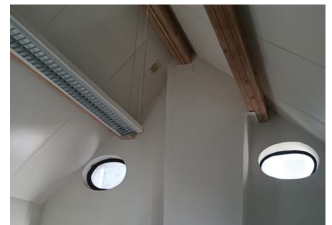
Figure 145. The purlin roof of the Pavilion
