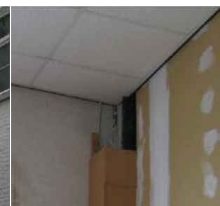
Figure 128. Steel column visible from the room next to the Sisters' chapel
