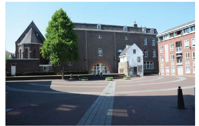
Figure 96. The Miséricorde plein, towards the complex
