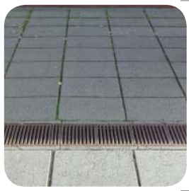
existing pavement in the main shopping street (2)
