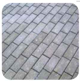
medium quality pavement connecting the key locations
