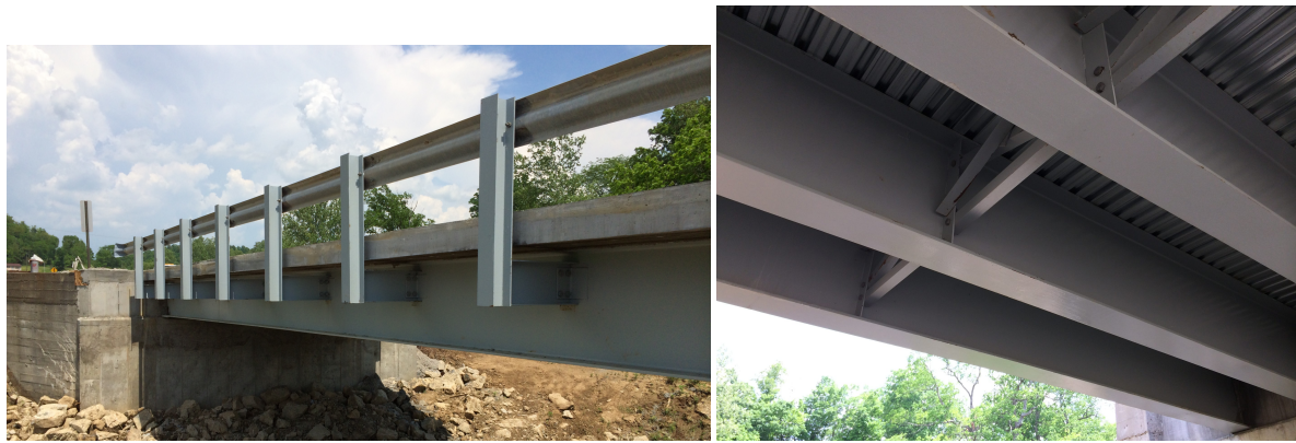
Figure 1.4: Reclaimed steel beams in new short span bridge in Ohio (Snyder, 2022)
