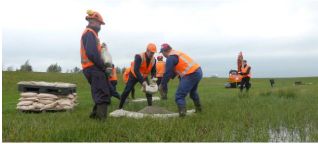
Figure 13: Containing sand boils (left) and constructing a soil berm (right)
