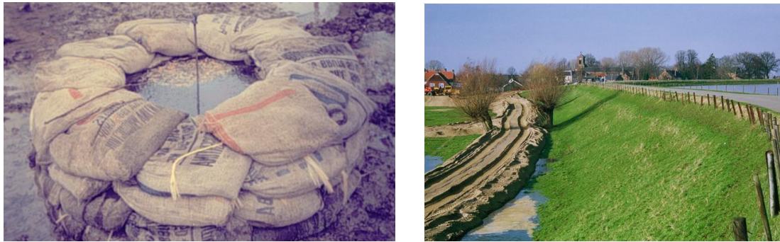
Figure 32: Containment of a sand boil (left: Dupuits) and filling a ditch at the toe of the dike (right: Waterschap Groot Salland)
