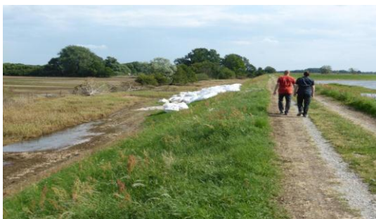
Figure 15: Placement error (E.J.C. Dupuits)
