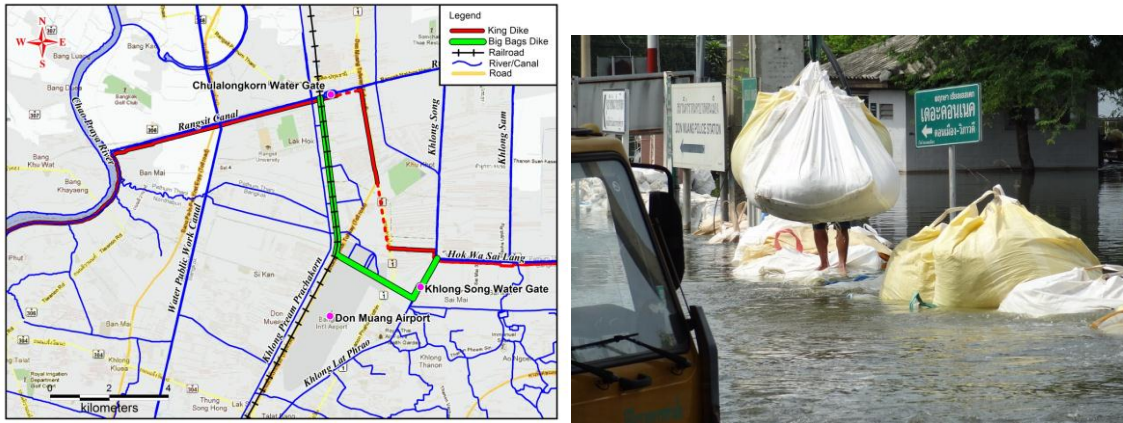
Figure 6: King dike Bangkok (left) and placement of big bags in gaps (right) [Jonkman]
