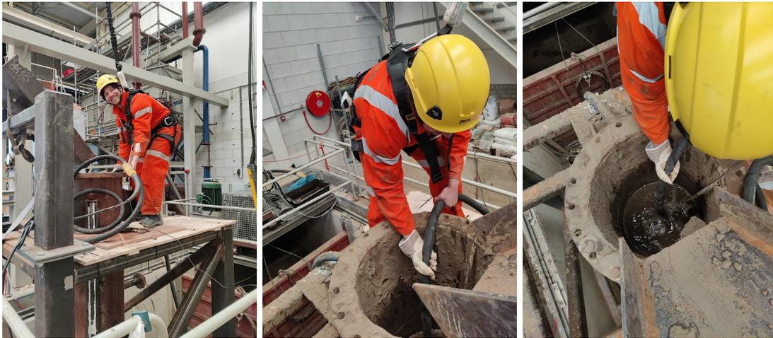
Figure 5.9: Needle compaction, note the safety harness and the platform
