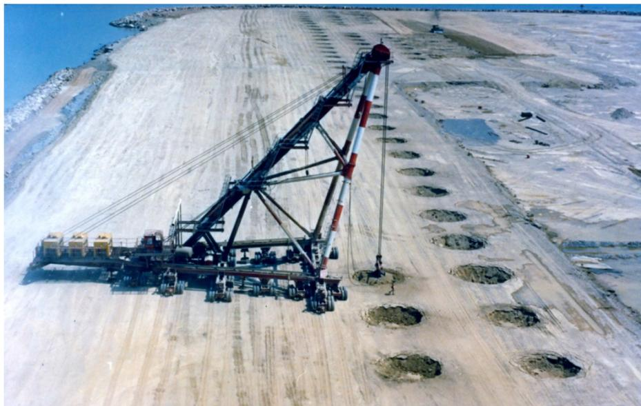
Figure 2.12: Menard's "Giga" compactor drops a 200 ton weight. (from Nicholson 2014, picture of Menard)
