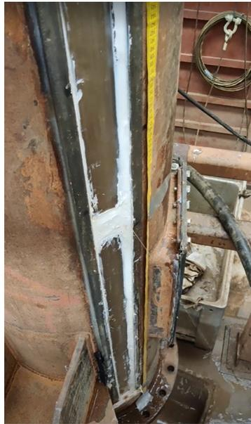
Figure 7.3: Leakage induced by gas pressure
