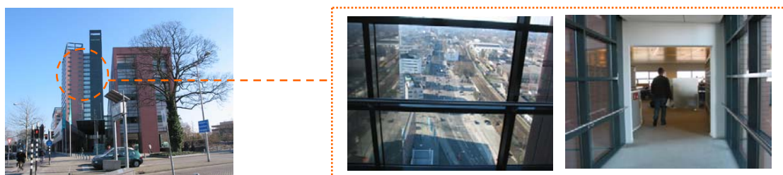
Fig 30 The connecting bridge elements: exterior and interior views
