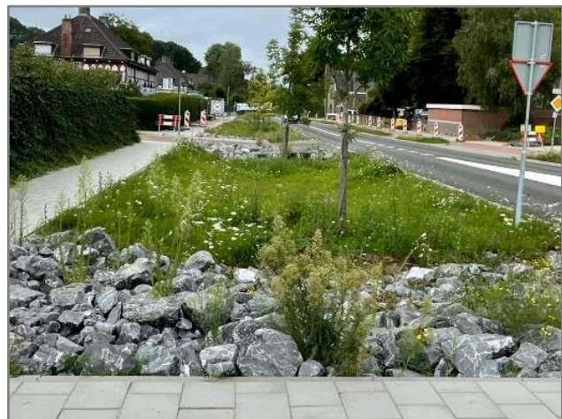
Figure 5 Rain garden between road and sidewalk. Heerlenseweg, Landgraaf. (Author's own picture).
