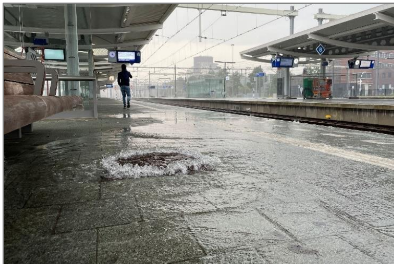
Figure 2 Overflowing sewers during an extreme summer rainstorm, on the 9 th of July 2023 in Zwolle, the Netherlands. (Author's own picture).
